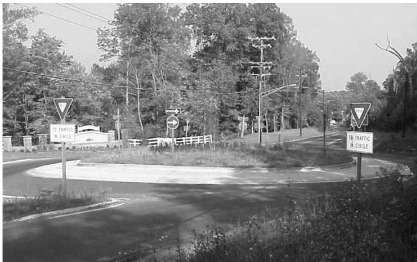
A modern roundabout, not to be confused with its less-safe predecessor, the
